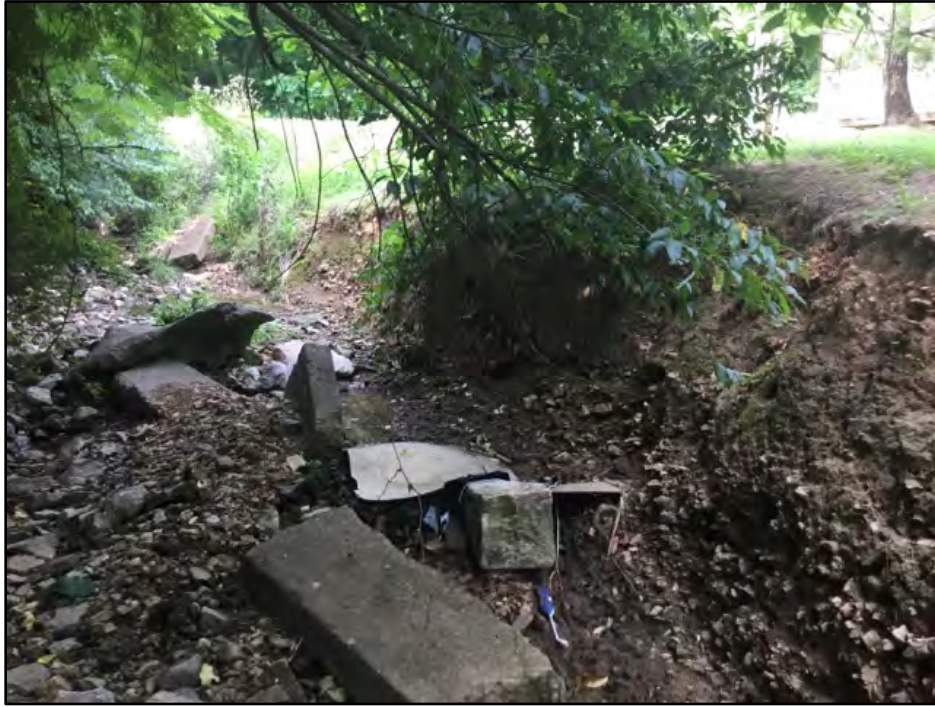
Photo 6 - View of the Erosion Site
