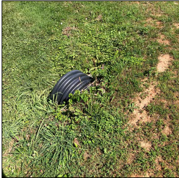
Photo 10 - View of Channel Alteration (Inlet)
