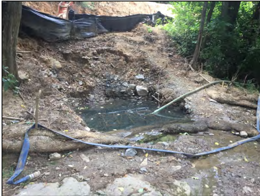
Photo 2 - View of Dewatering Activities
