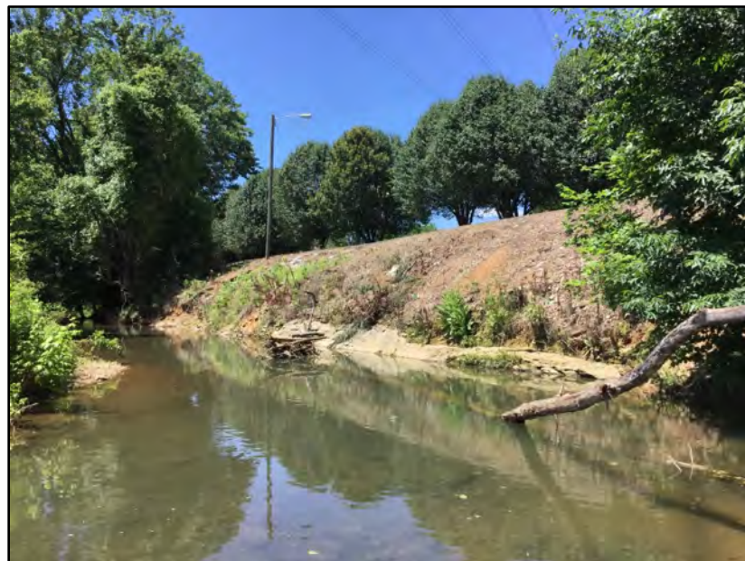
Photo 23 - View of Inadequate Buffer and Bare Bank
