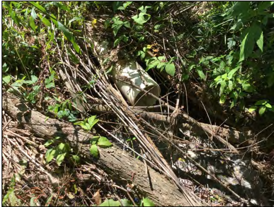
Photo 25 - View of the Pipe Outfall
