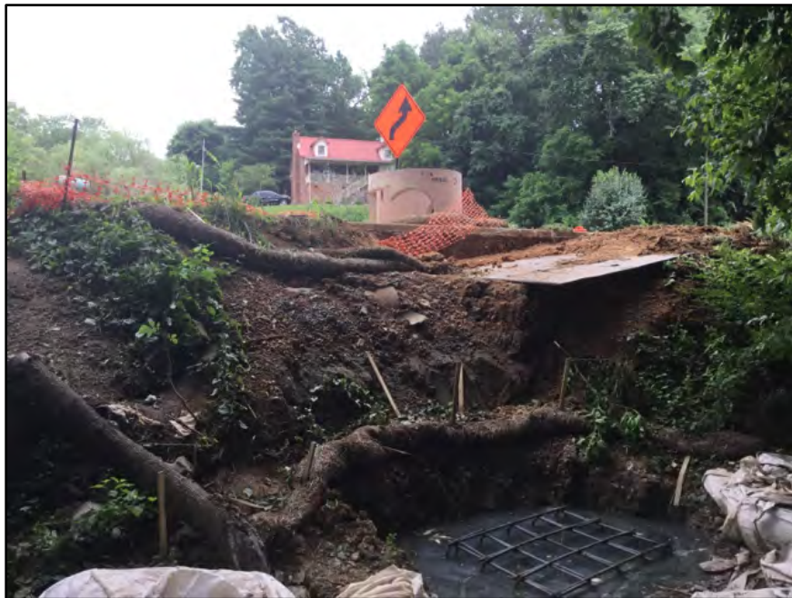
Photo 3 - View of In-Stream Construction
