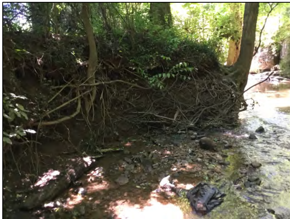
Photo 8 - View of Erosion Site
